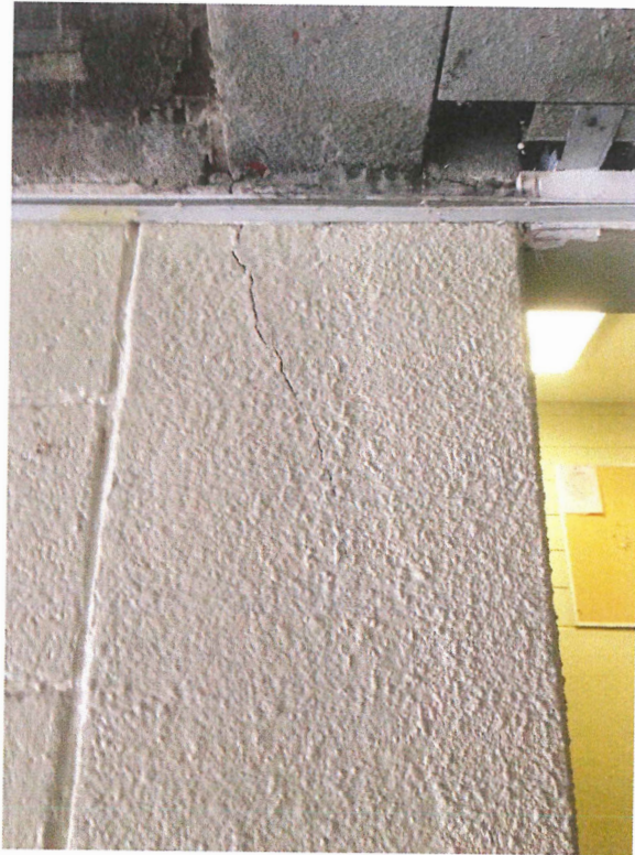
Damaged beam bearing
