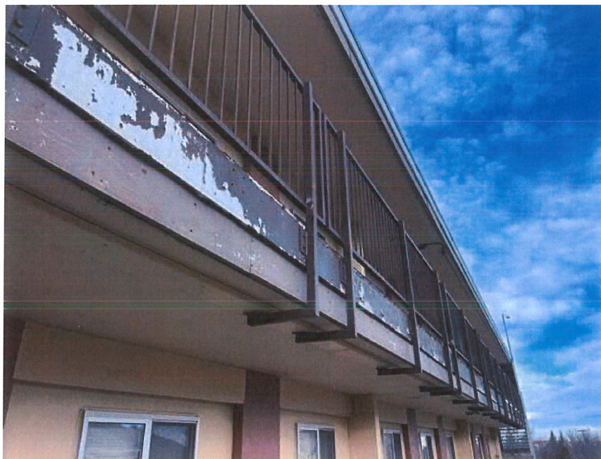
Photo-1: Walkway Handrails.
