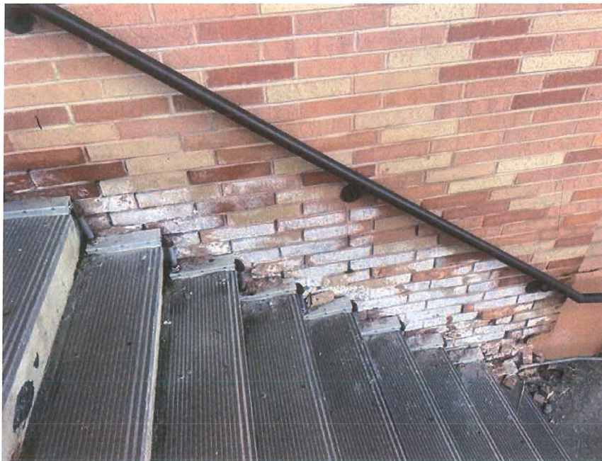
Photo-4: Damaged exterior brick at north-east.
