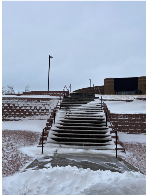
Stairs from Overflow
