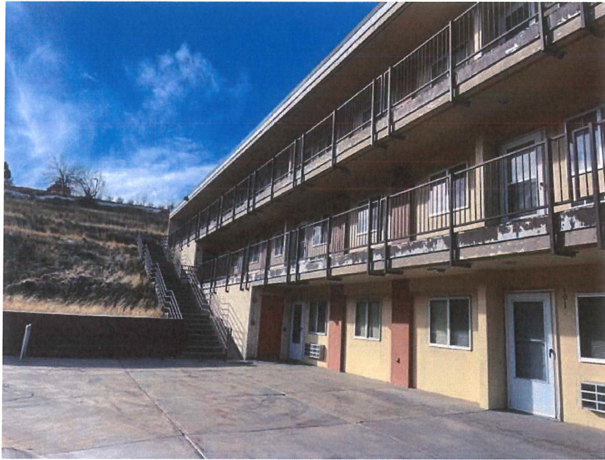
Photo-2: Exterior walkways at second and third floors.
