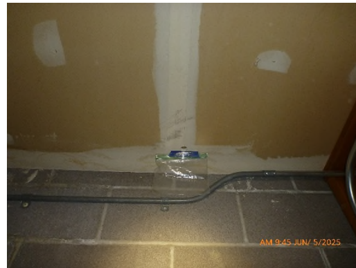
25-082-47 (Room #300 Storage Room)
