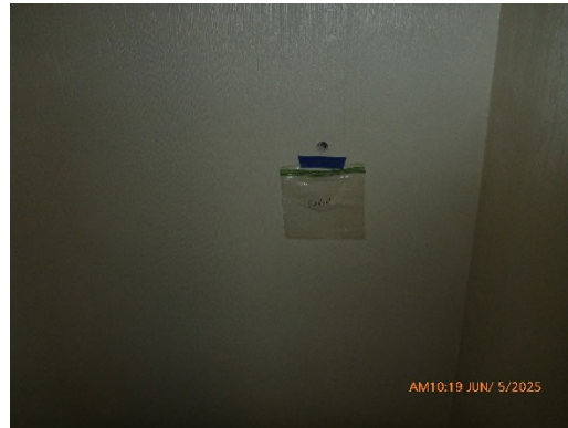
HA4-4 (Coat closet, Apt. #306)
