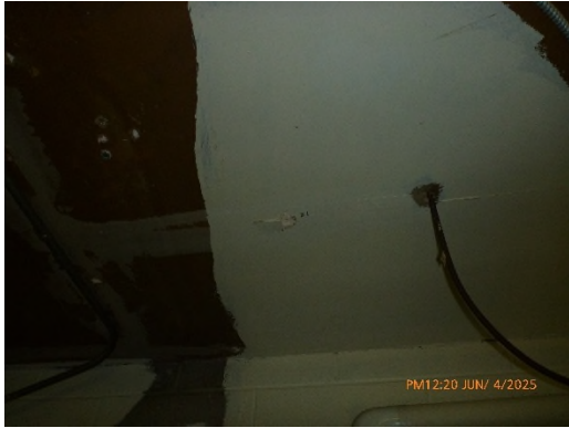
25-082-32 (SE Corner Boiler Room)
