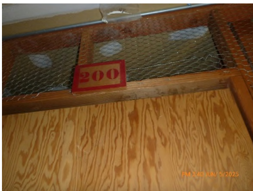
25-082-49 (2 nd Floor Storage Room)
