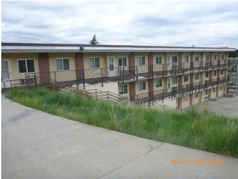
Wheeler Apartment Building (subject property) on the Casper Community College campus.
