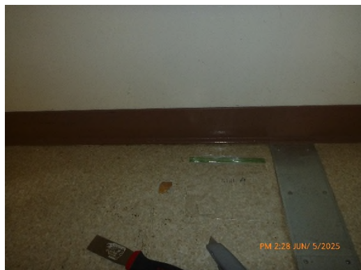
MM-19 (Laundry Room)
