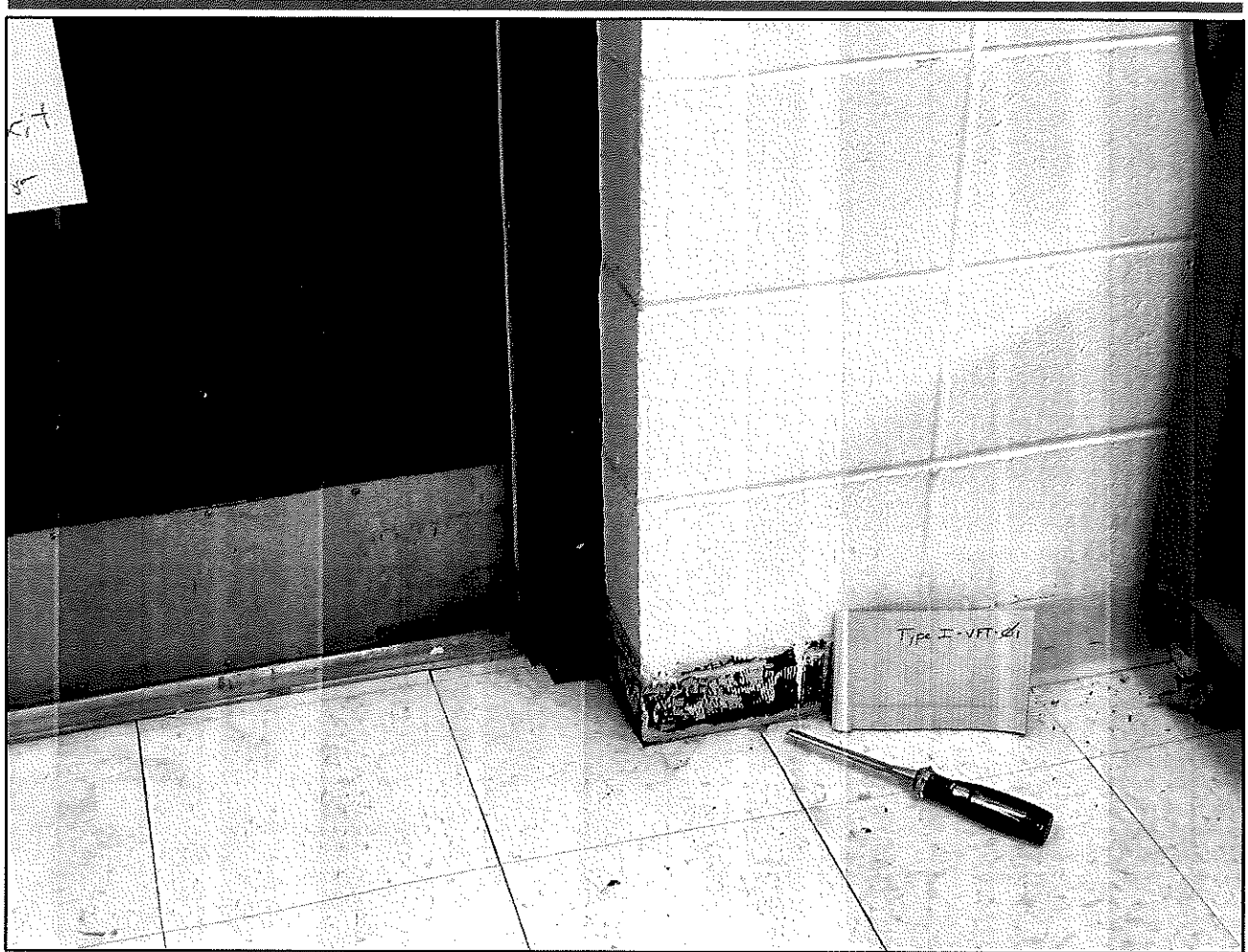
Photo 1. Room 106, sample location, Type I-VFT-01 (light tan 12"x12" vinyl floor tile).
