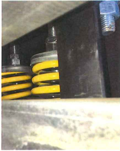
P2.4: Isolation Curb Springs at Section C
