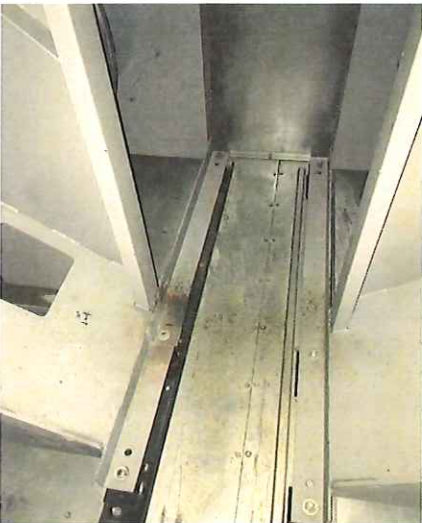
P4.4: Supply Fan #3 Blower Rail Repair - Welded on Steel Angle
