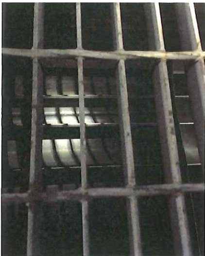
P3.4, 3.5, & 3.6: Supply Air Discharge Ducting Transition - Reduced Open Area, Turning Vanes, & Sound Attenuation
