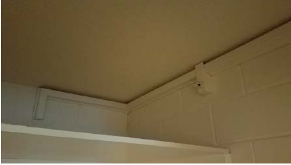
Photo of fire sprinkler line that must be protected during abatement
