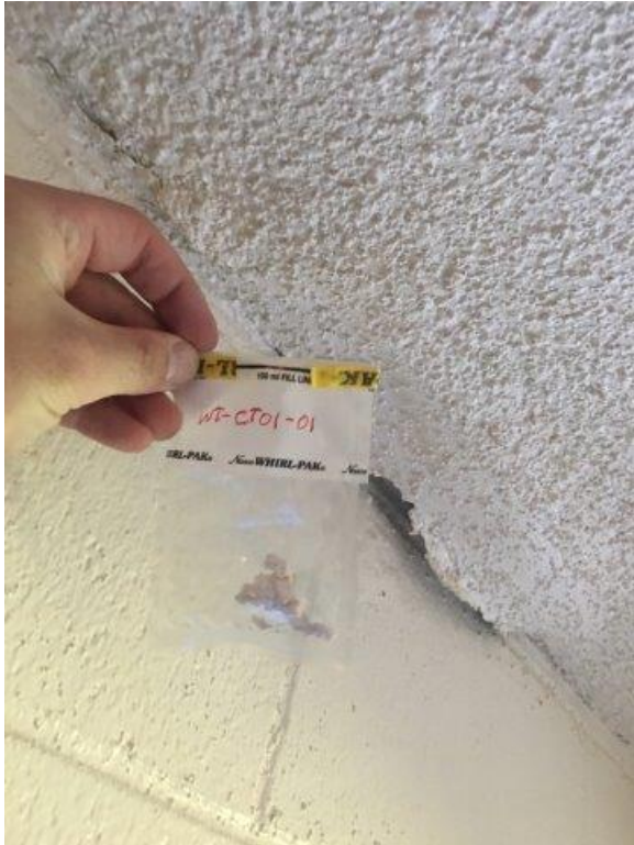
WT-CT01-01-Popcorn Ceiling Texture- Room 306, southwest corner-6% Chrysotile
