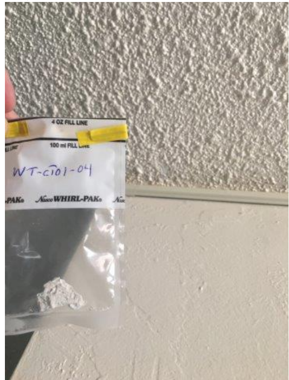
WT-CT01-04- Popcorn Ceiling Texture- Room 307, corner of kitchen and hallway-8% Chrysotile
