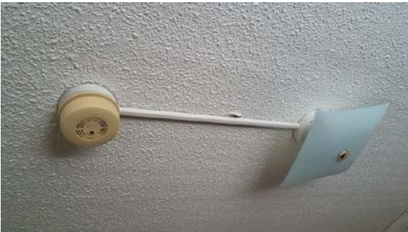
Photo of smoke alarm and light assembly that must be removed, cleaned and saved for reuse by Owner
